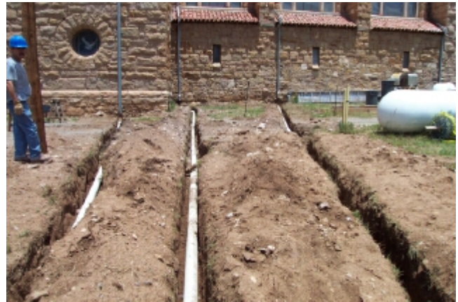
Brother David laying down new drainpipes.
