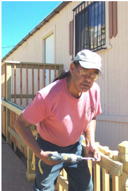
Bruce Klinekole building handicap ramp.
