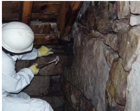
Harry Vasile repointing northeast interior wall.
