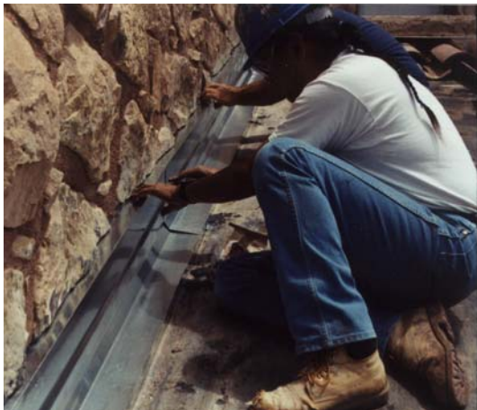
Tommy Spottedbird installing flashing.
