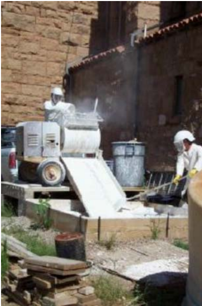
Brother Peter & Harry Vasile mixing lime-hydrate into putty mix.
