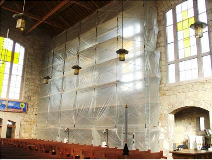
North wall interior being restored
