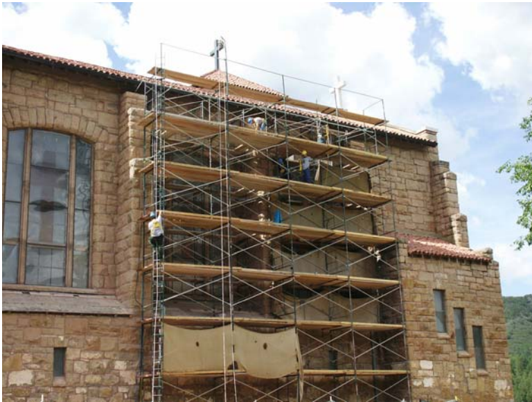
north wall restoration work underway
