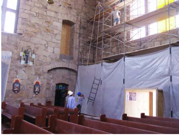
west wall scaffold being removed
