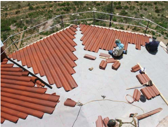
The crew from Smith Roofing, Inc. re-roofs the two sections of roof on the east end of the church, using Ludowici clay roof tiles and heavy duty copper flashing. KD Enterprises installed the new copper gutters and downspouts on the lower roof of the east end.
