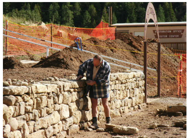
Completed portion of the wall
