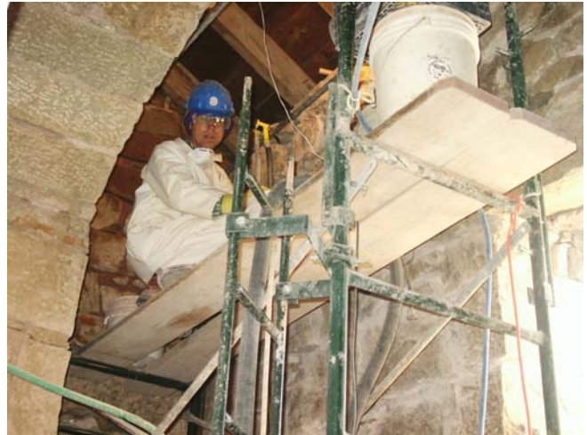
Brother David repointing in alcove
