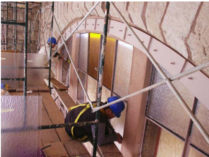
Bro. David and Arylis installing new window panels
