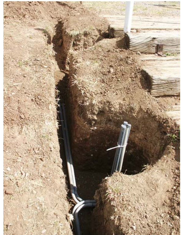
Restoration Crew installed conduit for electrical upgrade work.
