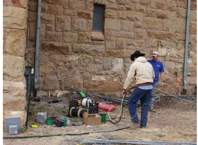
Shanti Electric crew running new electrical lines
