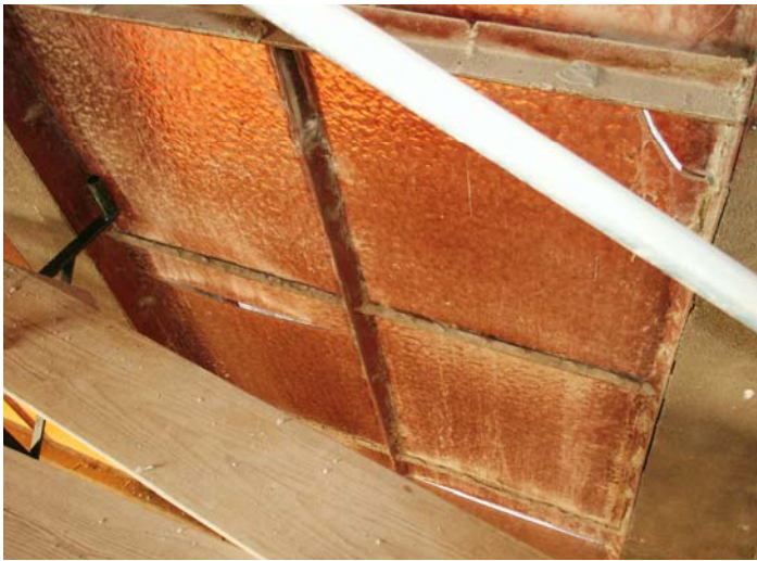
Closeup of west window before work began
