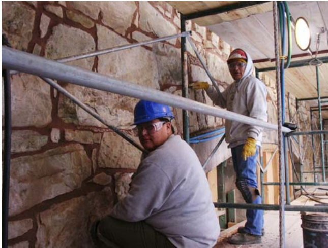
Arylis & Tommy repointing stonework
