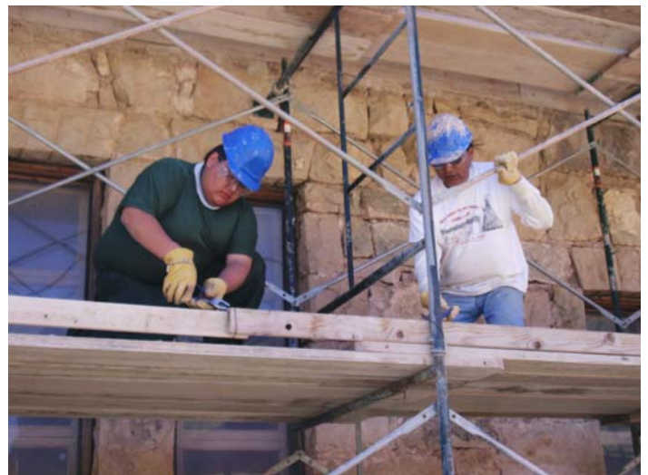
Arylis and Tommy setting up scaffolding outside.
