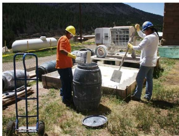
Restoration-trainee Walter and Tommy bring in the newly prepared lime putty for the mortar. The hydrated lime is being donated by the Chemical Lime Company.
