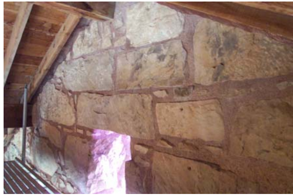
After: Repointing complete.
