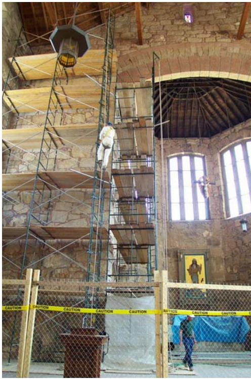
Brother David climbing scaffold ladder.
