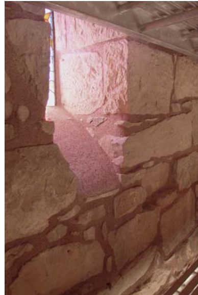
After: Rebuilding and repointing Completed.
