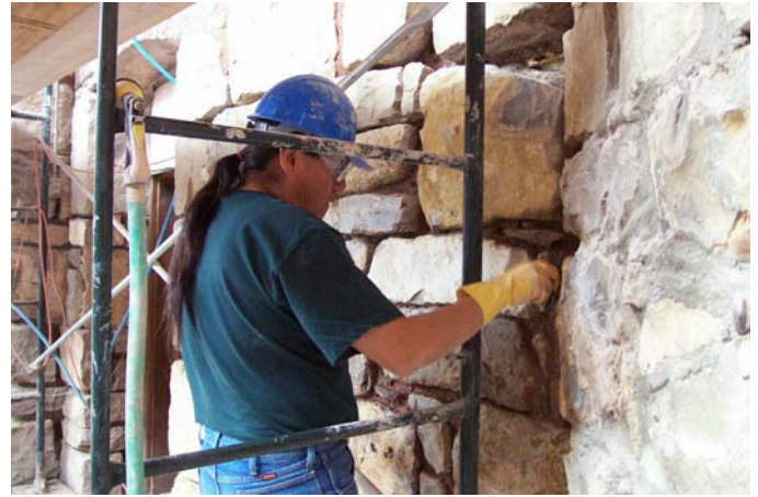
Tommy Spottedbird repointing north wall of sanctuary.
