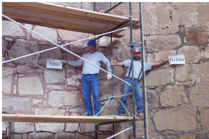
After: Rebuilding and repointing Completed.
