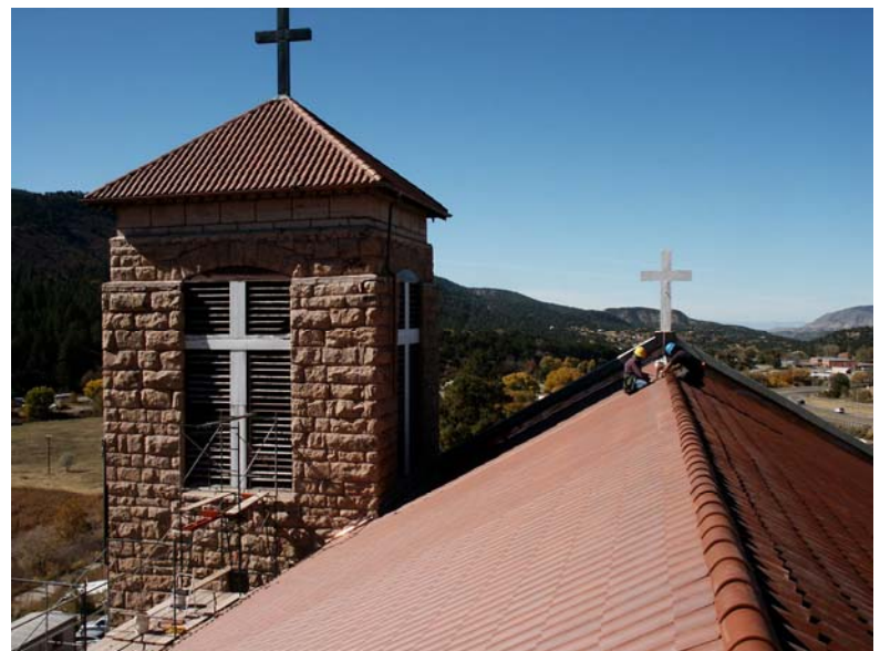
Finally the ridge cap goes on! Sam Sosa and Martin Pizarro are lining up the last few ridge tiles.
