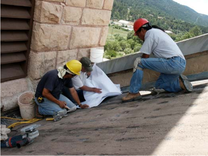
Architect Dale Zinn up on the roof to refigure plans.
