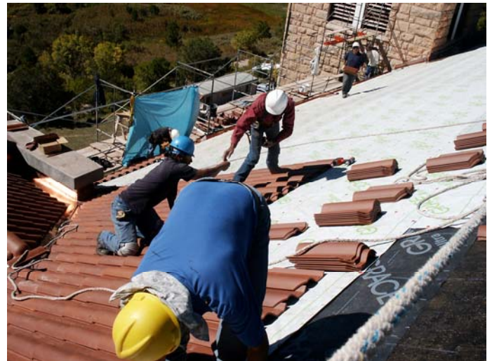
Our crew became great roofers!
