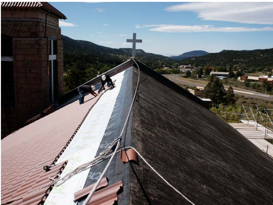
South side just about finished Robert Morgan aligning tile while Andres Ramirez screws them down.
