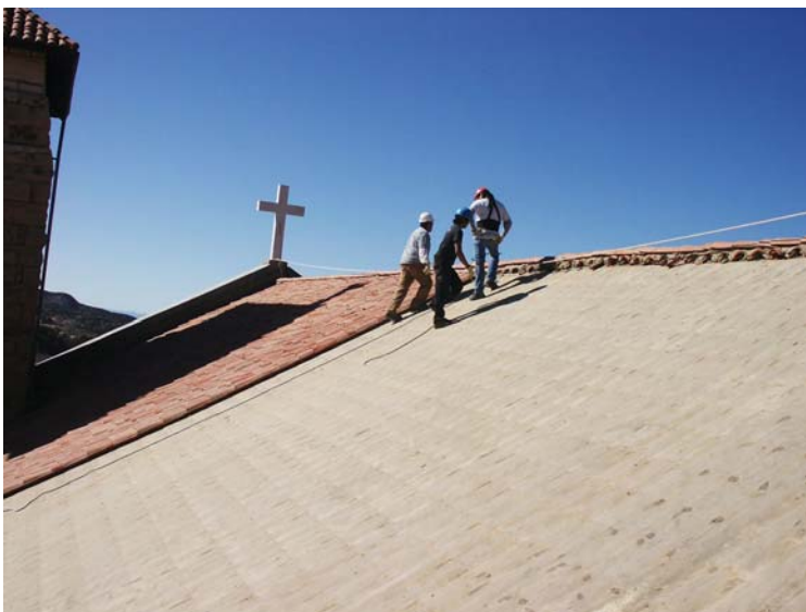
Arylis Chee and Lyle Magoosh helping Tommy Spottedbird remove the old tiles from the main roof.
