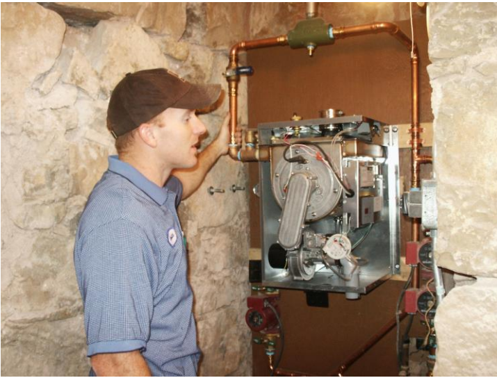
Josiah installing the new boiler unit.
