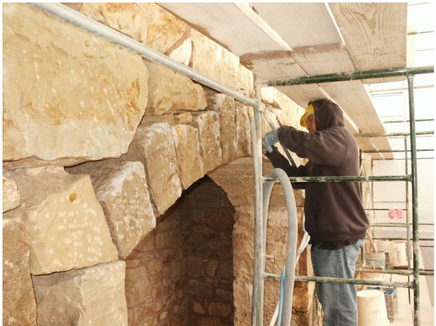
Nikona repointing alcove arch.
