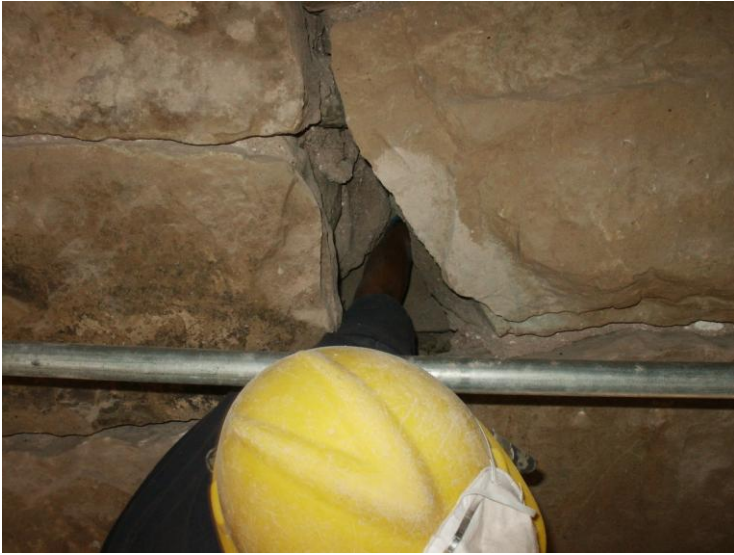
Sam preparing a deep void for repointing.
