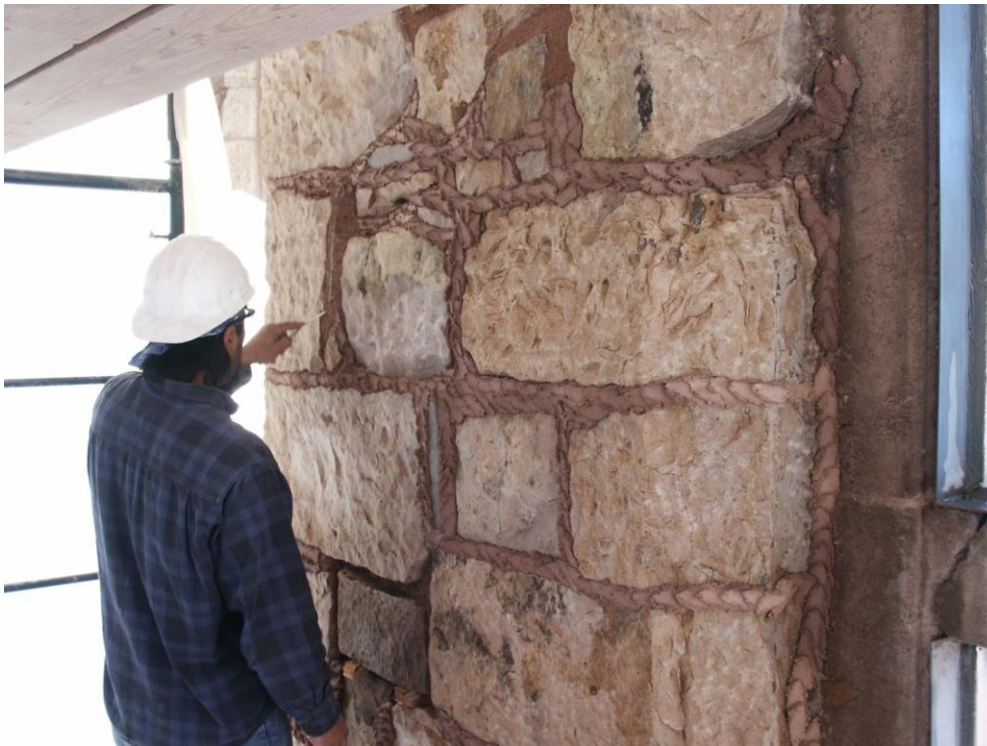
Sam using his new skills scrapping back the top coat, making it smooth and uniform.
