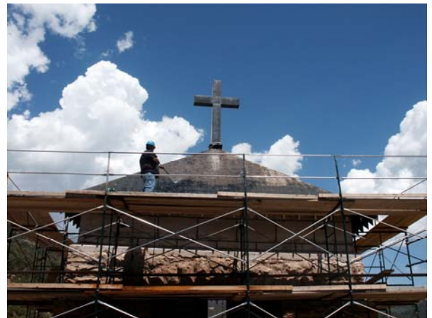
Arylis Chee power washing the bell tower roof
