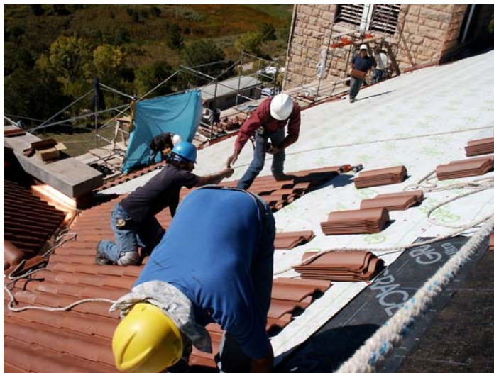
Roofing crew making progress
