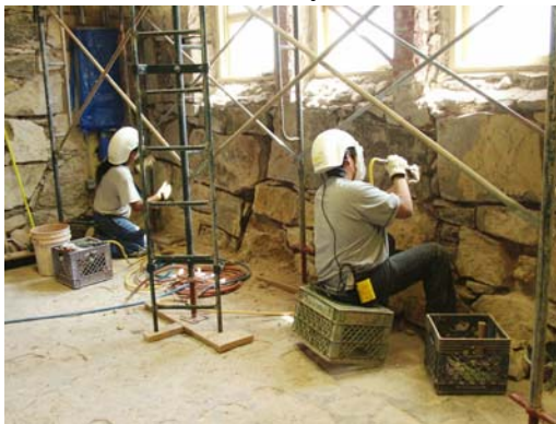
Removing deteriorated mortar
