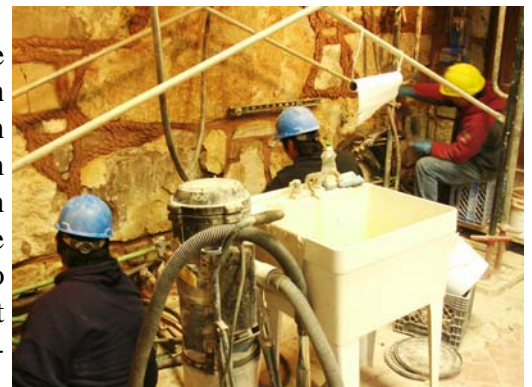
Repointing the stonework with lime mortar
