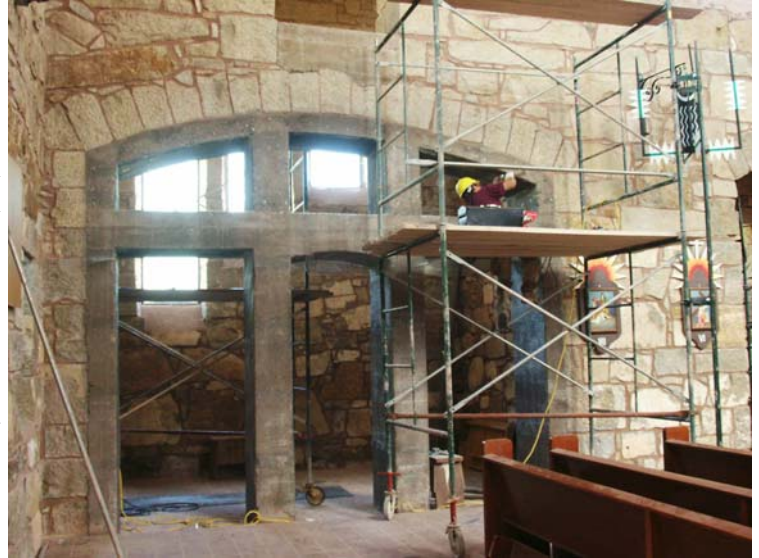
Martin Pizarro preparing to stucco staircase room entry.
