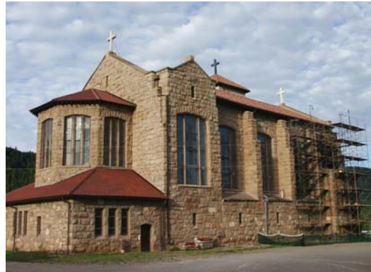
Scaffold on western end of north wall
