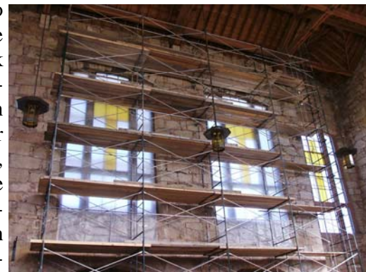
North wall interior
