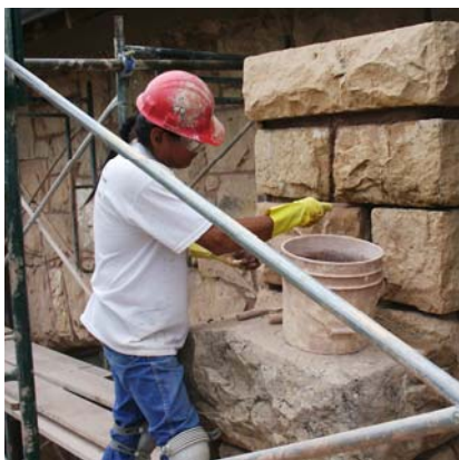
Tommy Spottedbird repointing
