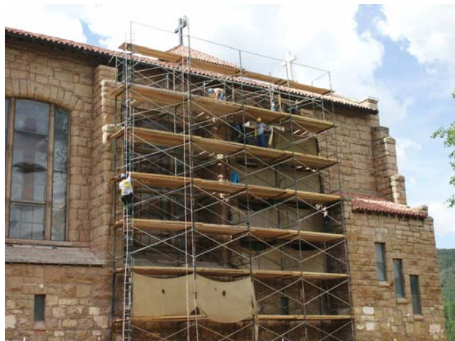
North wall exterior
