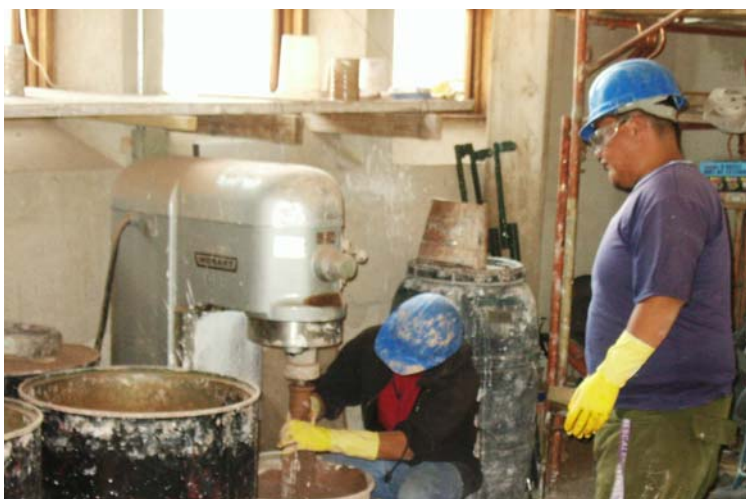
Arylis Chee instructing Nikona in the art of mixing mortar
