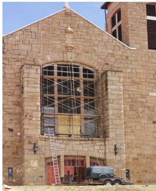
Ricky Jones sandblasting the frame
