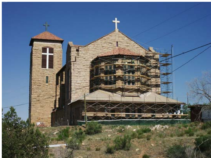
Summer 2004 work on apse exterior
